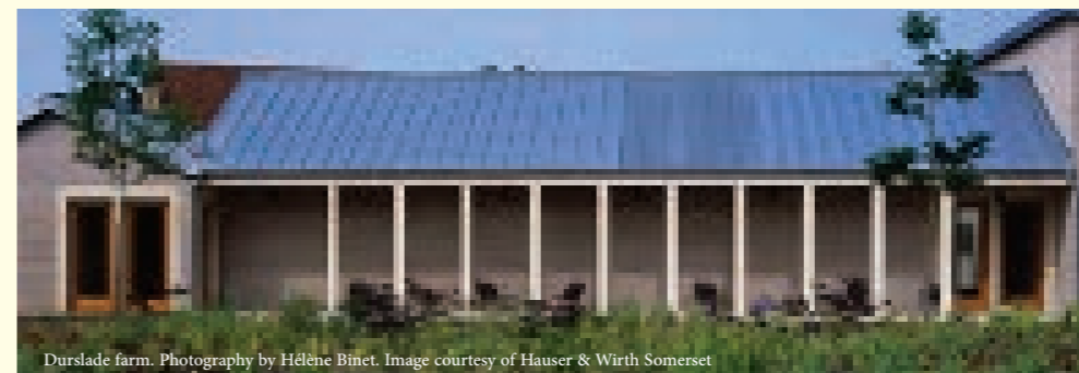
Durslade farm. Photography by Hélène Binet. Image courtesy of Hauser & Wirth Somerset
